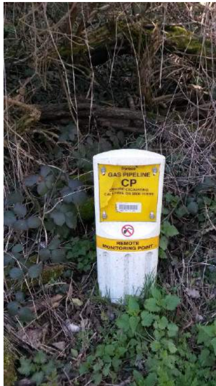
An existing marker post marking the Hemel Hempstead to Picketts high Pressure Gas Pipeline. This marker post is located within Phase 3 at the boundary of the land owned by Hertfordshire County Council and the land owned by Pouchen End Farm.
