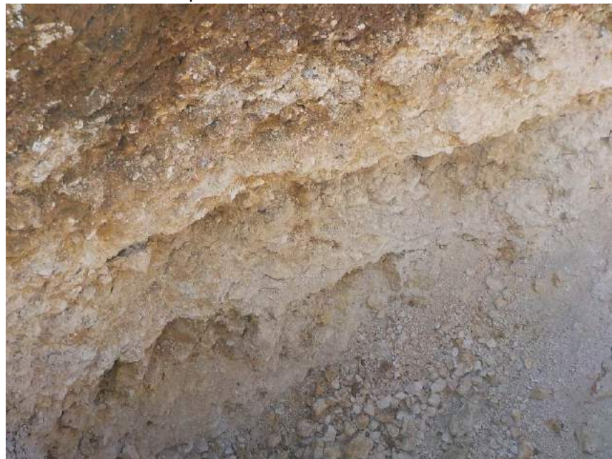
TP231 facing south. This was one of the trial pits within Phase 3 where grade C5 structured chalk was encountered.
