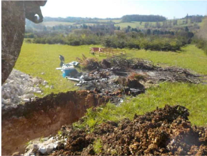
TP229 facing south. This trial pit was located to target a bonfire area which also contained rusted metallic cans. Following chemical testing of soils at 0.20 and 0.50mbgl, no exceedances in guideline acceptance criteria was encountered.
