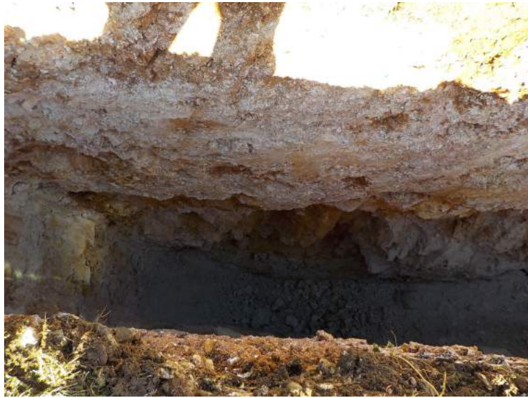
TP304 facing north. This was the only trial pit excavated during the Autumn 2016 Ground Investigation where structured chalk was encountered.
