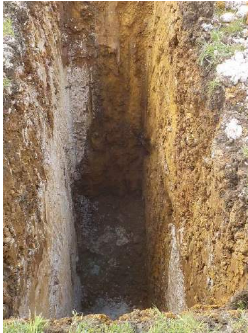
TP215 facing south
