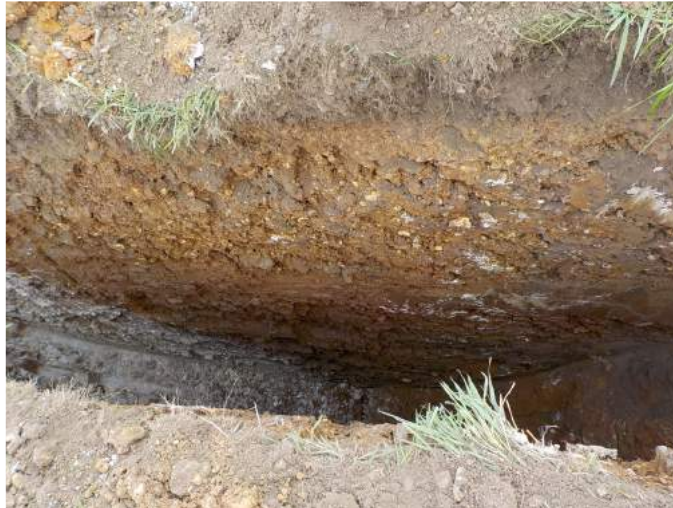
TP327 facing south
