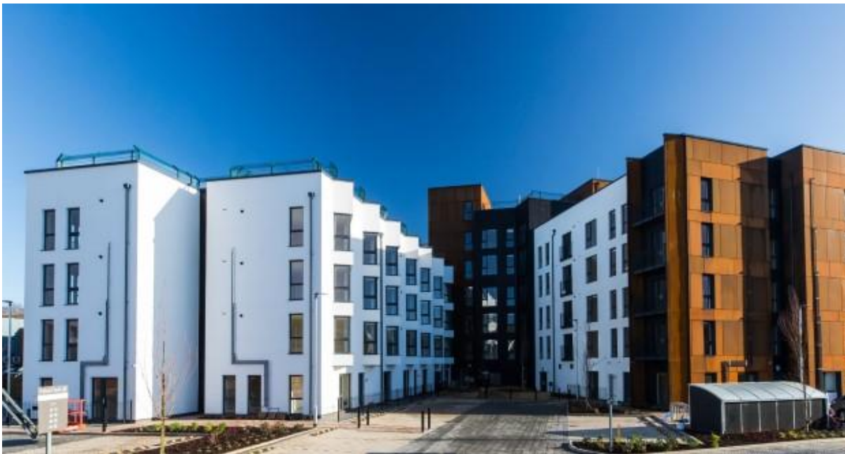
Kylina Court in Hemel Hempstead - providing 79 homes for social rent
