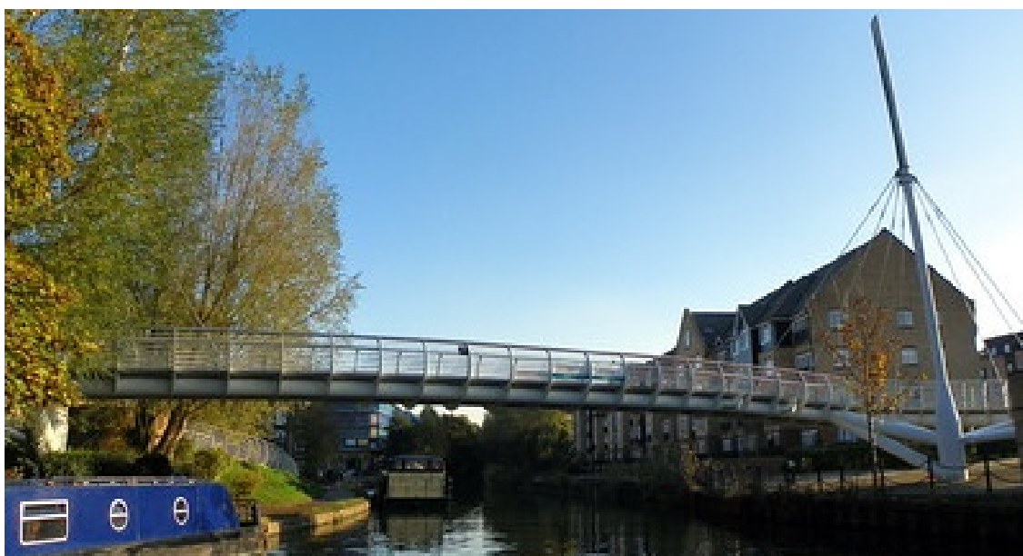
Figure 2-3: Apsley canal and cycle bridge
